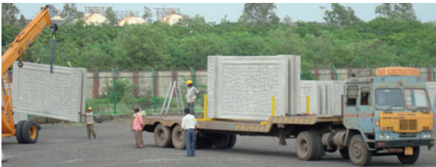
Transporting panels to fence line
