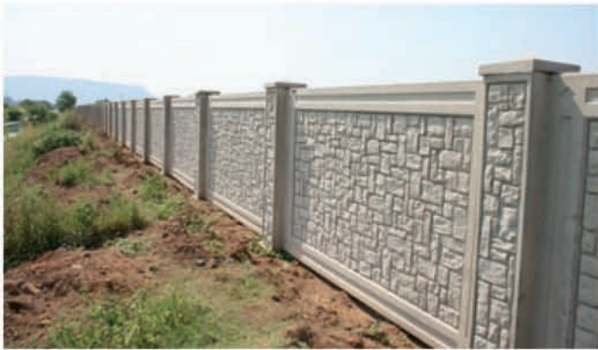
Installed boundary wall
