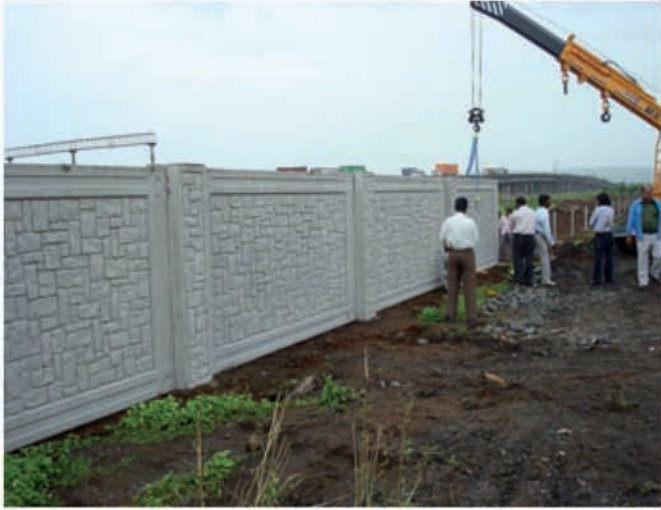
Commencement of installation
